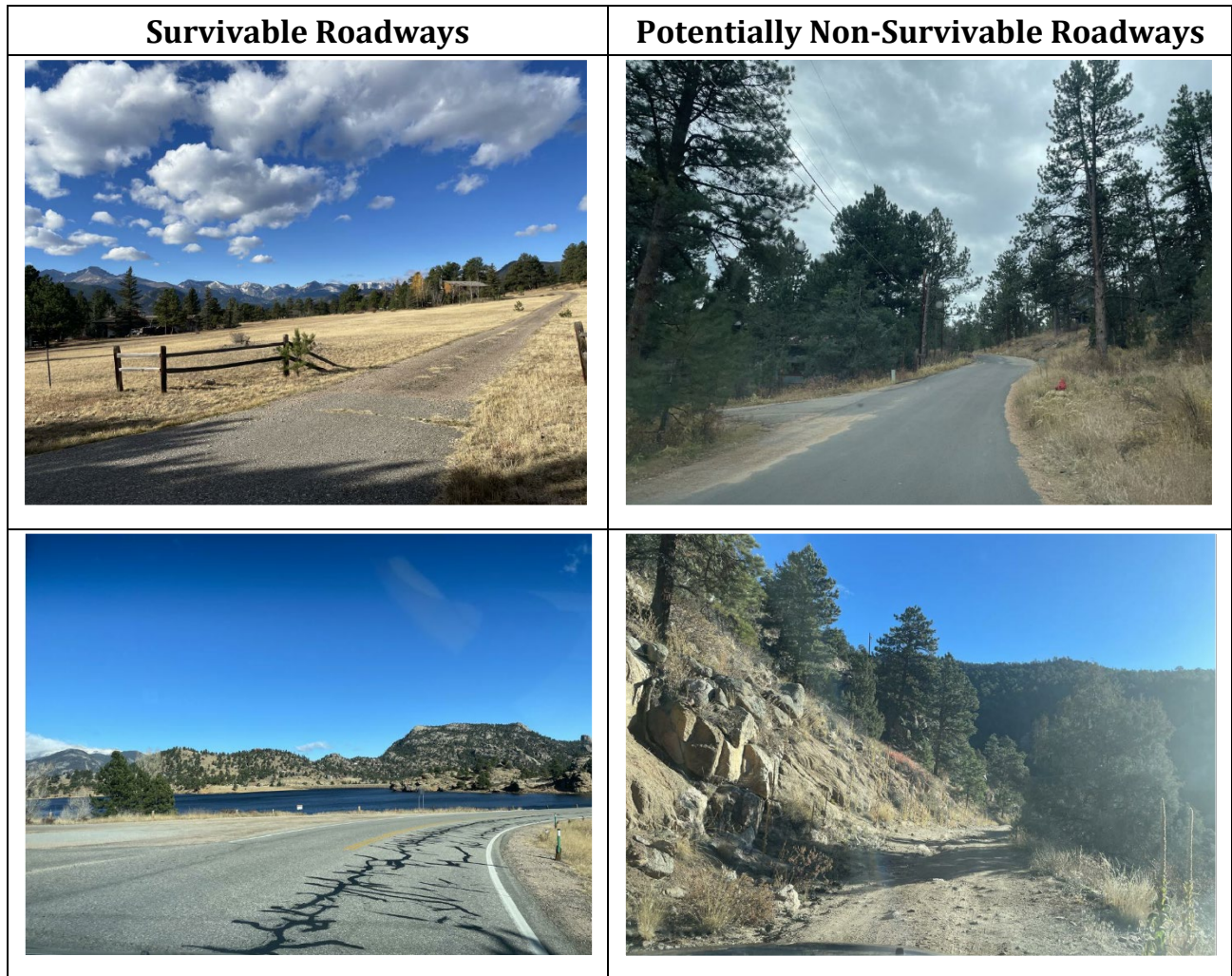
Figure 8.a.11. Some roads in the Estes Valley Fire Protection District have been well mitigated by removing tall trees and saplings, removing limbs on the remaining trees, and keeping grass mowed (left images). Other roads could experience potentially non-survivable conditions because they are lined by thick forests that have an abundance of ladder fuels (right images). Photo credits: The Ember Alliance.
