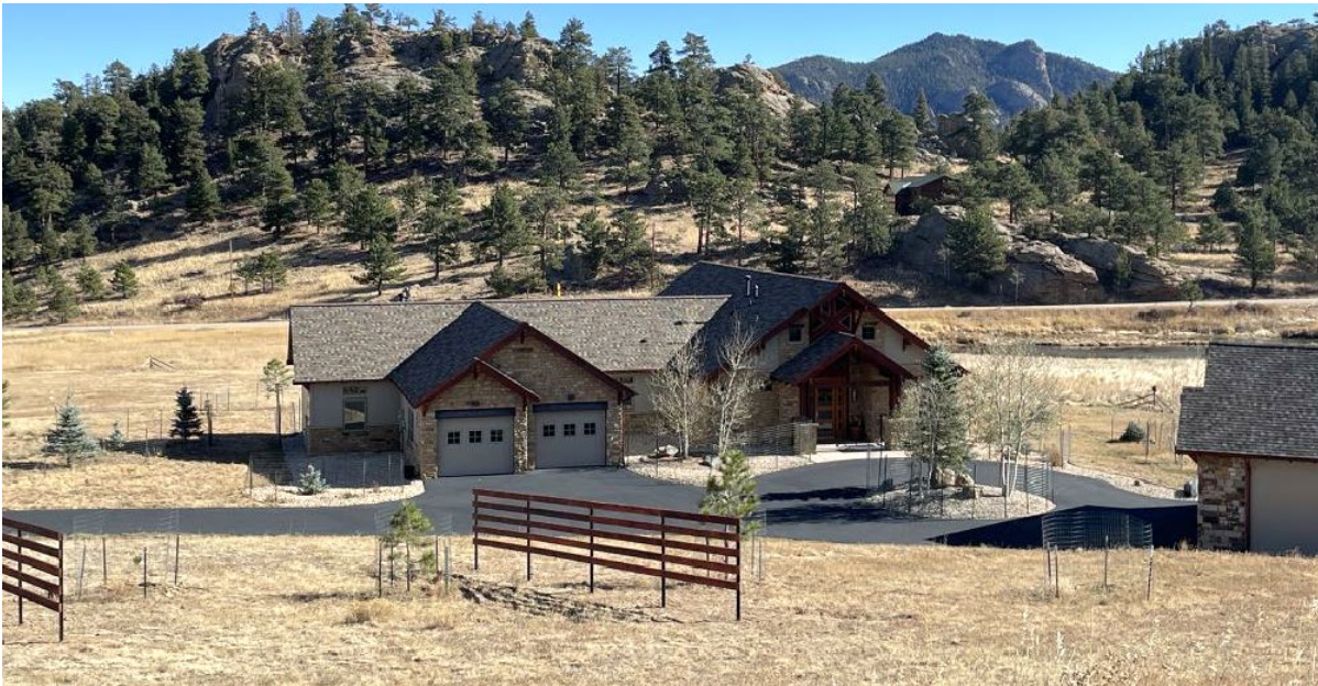
Top two photos: Tall grass and shrubs, tight crown space, and dense ladder fuels could endanger these upslope homes due to radiant and convective heating and short-range embers during a wildfire. Bottom two photos: Trees and shrubs near the homes are thinned, there is a 5-foot noncombustible zone around the structures, and the grass is mowed, making these homes more defensible and resistant to fire. Photos credits: The Ember Alliance.
