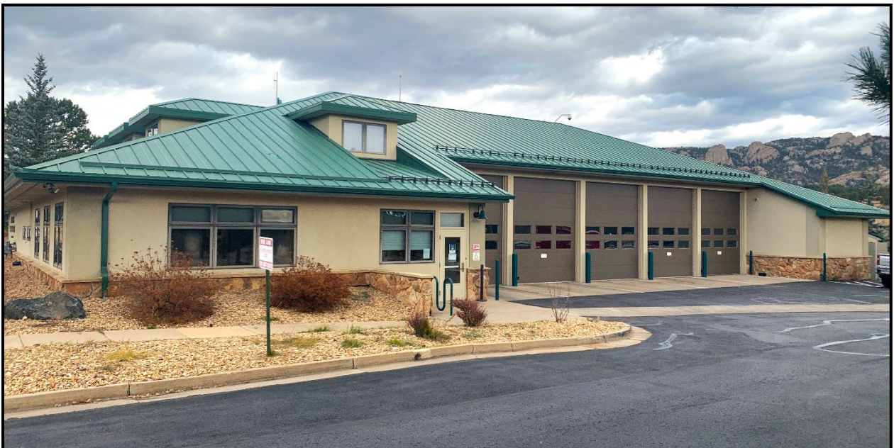
Station 1, Dannels Fire Stations, headquarters for the Estes Valley Fire Protection District. Photo credit: The Ember Alliance.
